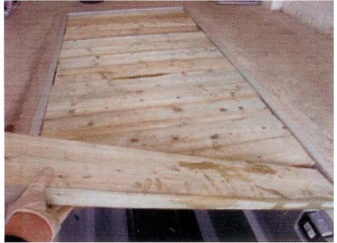
**14** Once the concrete is dry, measure across the top recess to find the length of the boards needed for the cover. Take  $\frac{1}{2}$  in (13mm) off this measurement to allow the boards to be easily removed. Mech-Mate recommends  $2\frac{1}{4}$  in (60mm) by 12in (300mm) boards. Very light cars could be safely driven over 2in (50 mm) boards (as in the pictures).
