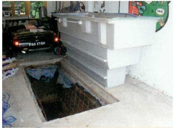
**8** With three assistants, carry the pit to the hole. Wear gloves to protect from glassfibre splinters. Loop rope at the front and back of the pit and, with a person at each corner, lower it into the hole. Check the fit and mark any tight spots. Pull the pit out and place it next to the hole - it's better to know the pit is going to fit before you've mixed up any concrete.
