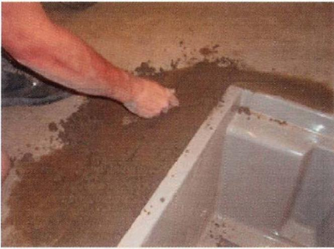
**13** Check all the electrics work, then apply silicone sealant to make the wiring holes watertight. Leave the silicone to dry for two or three hours and then make up another firm concrete mix. Pour in, taking care not to spill concrete into the pit. Finish off the concrete with a trowel, forming a slight slope to stop water getting into the pit.
