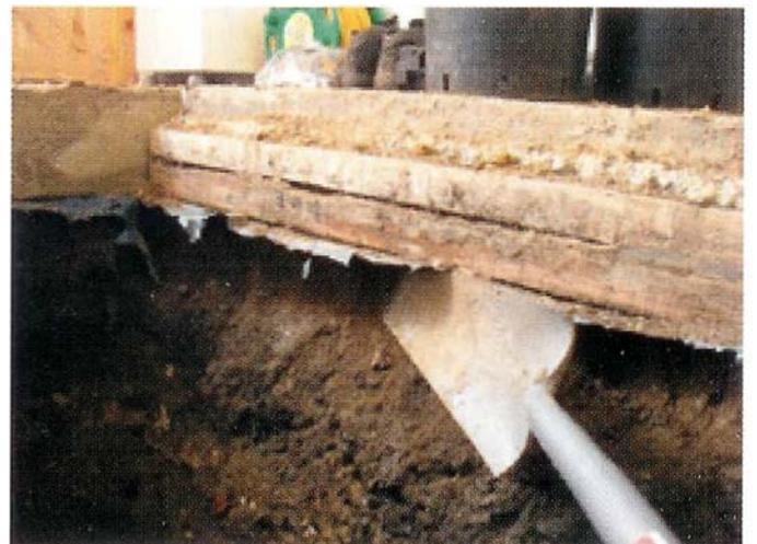
**4** Dig out a shallow channel in the hard-packed earth under the concrete floor. This allows the concrete that will be added later to flow in and add strength and support to the floor. At the base of the hole a similar channel should be dug into the walls. This helps to 'lock' the base of the pit in the concrete.
