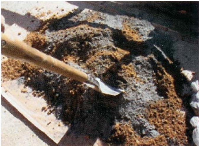
**9** Carry out any necessary adjustments to the hole and make up a wet concrete mix. Pour this mix into the hole to a depth of 4in (100mm). The 8ft (2.5m) long pit pictured here needed 220lbs (100kg) of ballast and two bags of cement. Mark off 4in (100mm) on a long piece of baton and push it into the concrete to check the depth.
