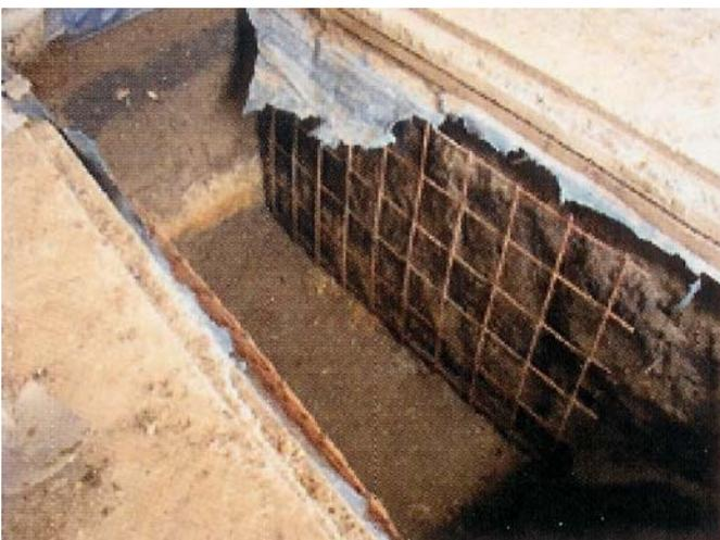
**5** Measure from the base of the hole up to six inches (150mm) beneath the existing floor level. Now measure the length of the walls. Mark these two measurements onto the steel reinforcement mesh and cut out using a grinder. You'll need two of these reinforcement panels, one for each side. Position both against the walls of the hole.
