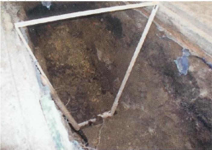
**3** As you dig out the hole, check it regularly with your wooden templates. When you think enough earth has been removed, walk the end profile template through the hole. If any part of the template catches, mark the area and scrape off the excess earth before walking the template through again.
