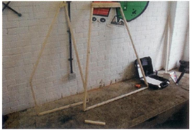
**2** Make up a template that matches the end profile of the pit and another that follows the angle of the steps. Use pieces of 1 in x 1/2 in (25mm x 13mm) baton. These templates need to be exactly the same shape as the glassfibre pit but 4in (100mm) bigger all round. Ten minutes spent making these will save you a lot of unnecessary digging.
