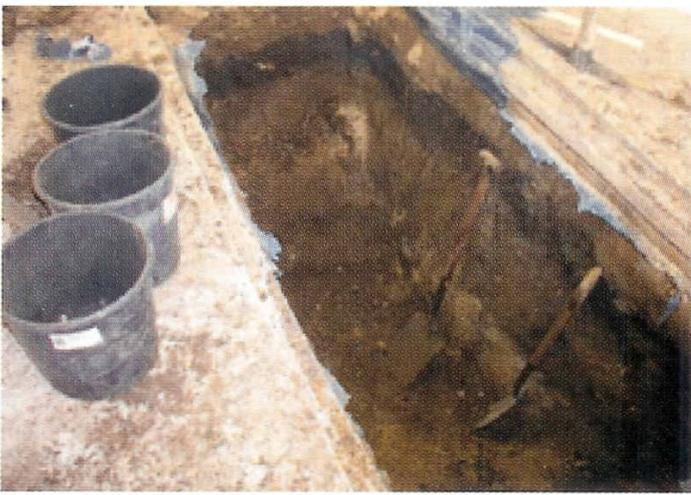
**1** Decide where you want the pit (see *Afraid To Ask*). If you are installing the pit in an existing garage, mark out the hole and cut through the concrete with a stone-cutting, disc-equipped grinder. Break the concrete out with a sledge hammer. The earth can be removed with a mini-digger, but you'll need buckets and a shovel for the lower reaches.
