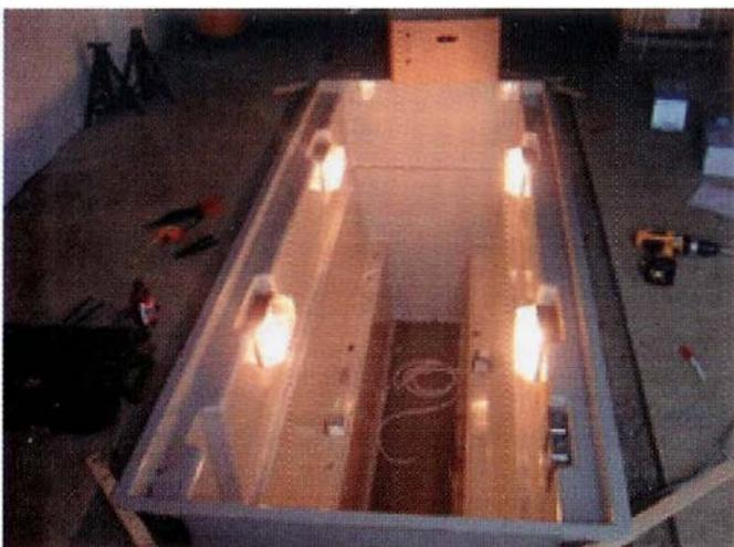
**11** Leave the pit overnight (12 hours minimum) to let the base harden. Make up a firm concrete mix and pour down the sides of the pit until it's 2in (50 mm) beneath the first ledge. Follow this with a wet mix around the ledge. Work the concrete down with baton and repeat as per the diagram to 2in (50mm) below the level of the wiring conduit.
