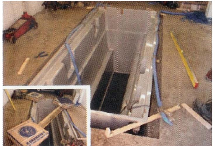
**10** With three assistants, lower the pit into the hole. The corners should be supported on lengths of ½ in (13mm) baton. This lifts the pit off the floor and will stop water running into it when it's in use. Climb into the pit to help it bed down in the concrete. Use planks and weights to help hold the pit in place while the concrete is drying (inset).
