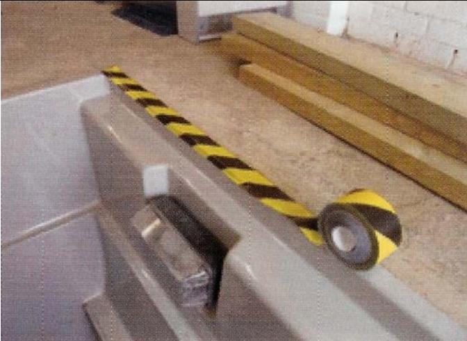
**15** Clean up any cement overspill and then apply safety tape to the edge of the pit. Extending the safety tape in front of the pit by a few feet makes lining up your car much easier. The concrete will need two days to harden fully, so don't be tempted to drive over the pit until then.
